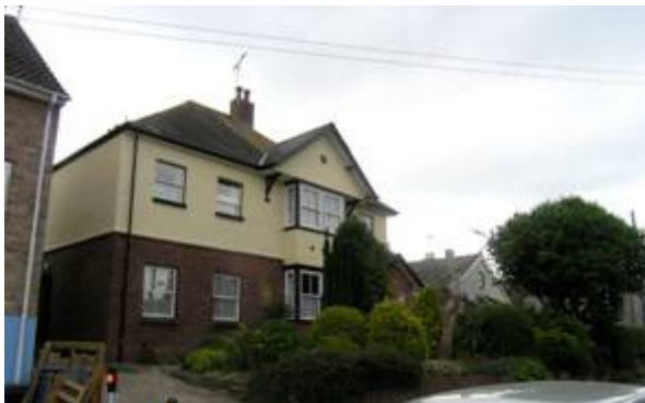
Figure 99: Suburban villa on Mill Lane.
