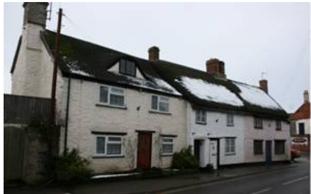
Figure 16: Ring Street historic plots; from right to left: Runaways Cottage, The Thatched Cottage and Birdseye Cottage.
