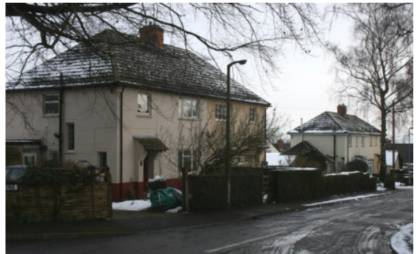
Figure 61: View east along Park Road showing mid 20 th century semi-detached houses.
