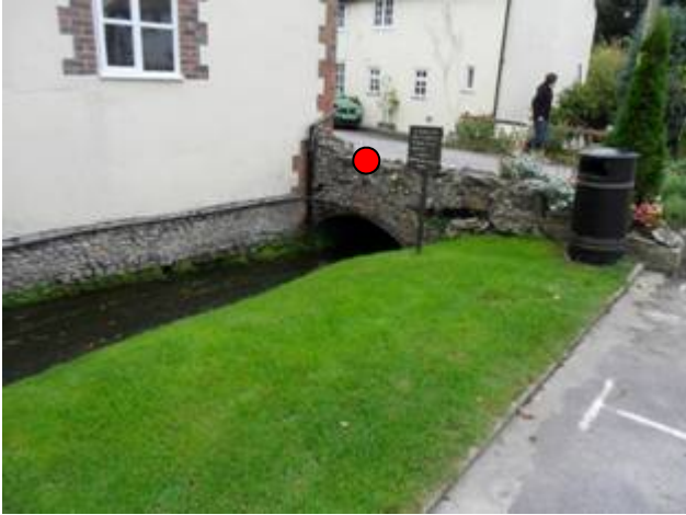
Take sample from bridge, u/s side and mid-channel
