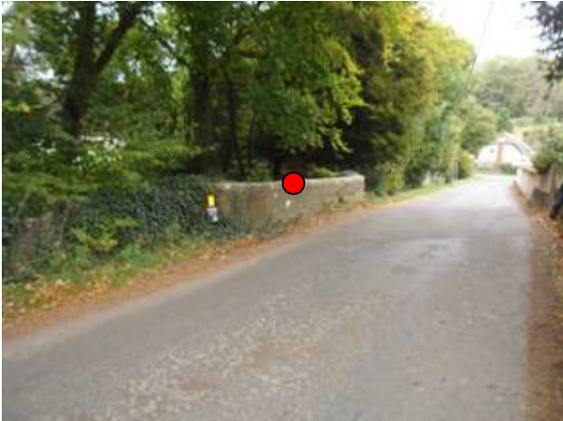
Take sample from bridge, u/s side and slightly towards the left hand side of the bridge span
