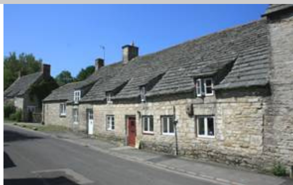
Figure 52: Early 18th century cottages, 50 West Street.
