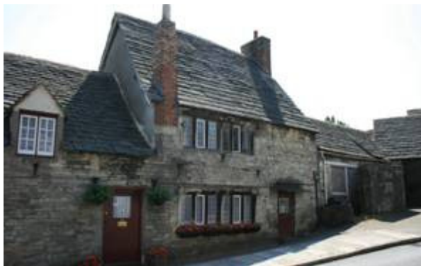
Figure 13: Uvedale's House, 17-21 East Street (built circa 1575).
