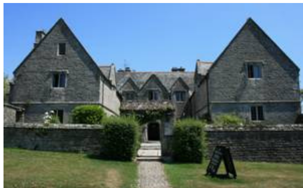
Figure 14: Morton's House, East Street (built circa 1600).
