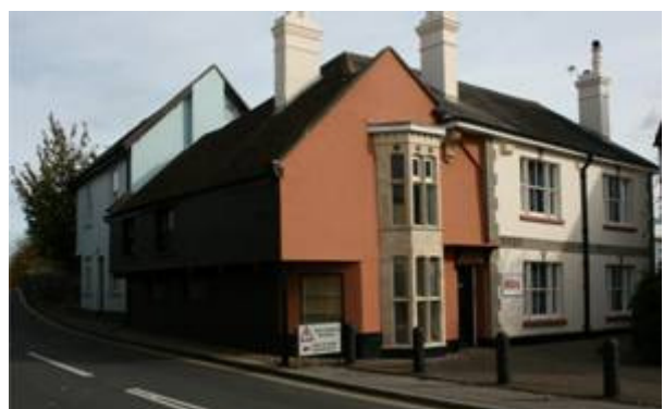
Figure 23: The Chandlery on Bridge Street. 18th century re-facing of a late medieval building.
