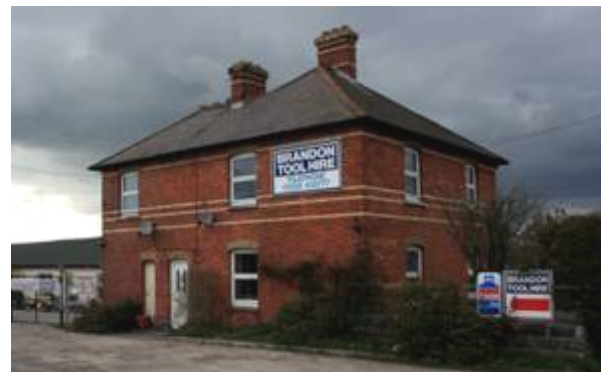
Figure 89: Pines House; the former matron's lodge for the Victorian Isolation Hospital, Shaftesbury Lane
