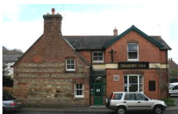
Figure 78: The Damory Oak Inn, with a 19 th century or earlier north wing on the left of the picture.
