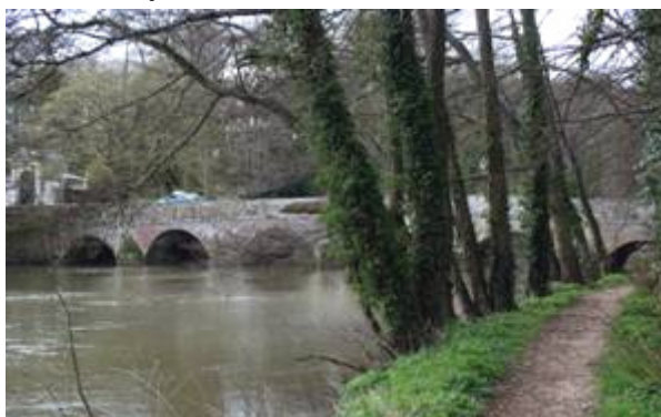
Figure 48: View west of Blandford Bridge
