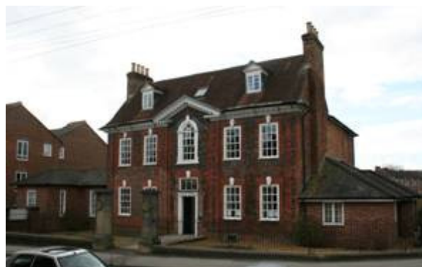
Figure 18: Eagle House, White Cliff Mill Street
