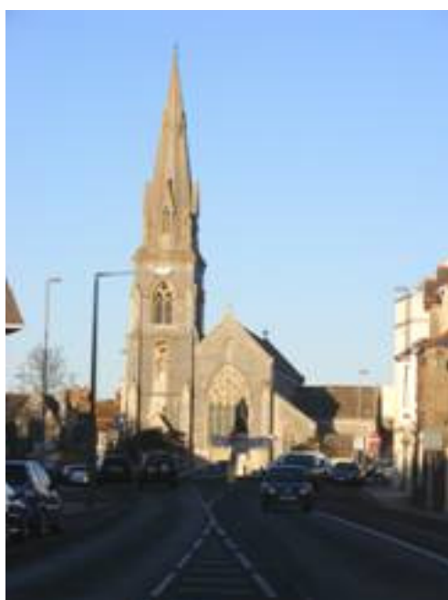
Figure 88: St John's Church
