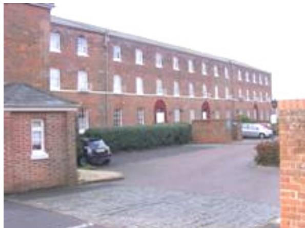
Figure 47: Former Weymouth barracks
