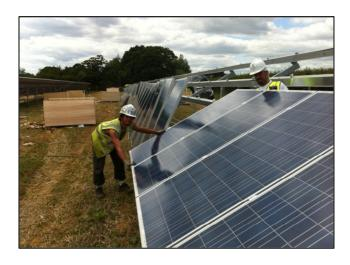
The system, designed by ANESCO, comprises 7,868 polycrystalline solar PV panels, arranged in in thirty two rows up to 165 metres long, generating DC power connected to a new 7.5MVA Primary Substation built for SSE Power Distribution, which 'steps up' the AC electricity from 11kV to 33kV
