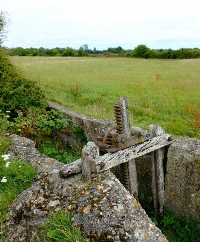
Figure 7.1: A surviving sluice in Stinsford water meadows
