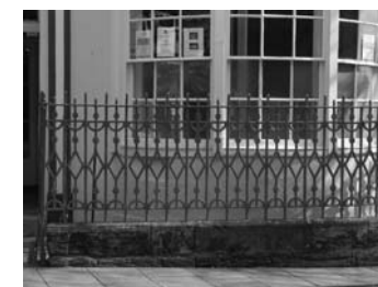
Fig.45 Iron railings, Digby Estate Office
