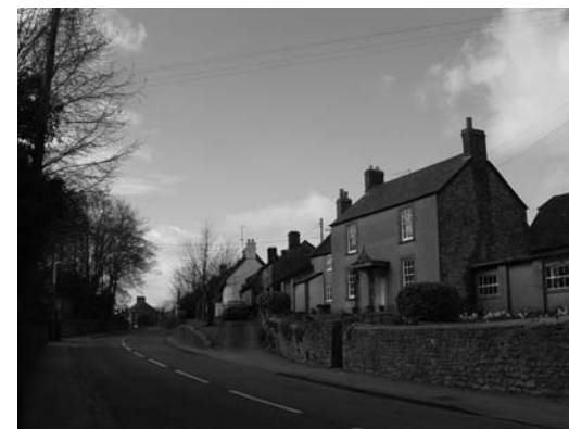
Fig.75 Building details, Yeovil Road
