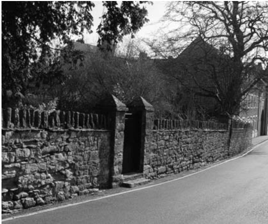
Fig.41 Boundary Walls, Hospital Lane
