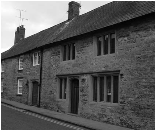
Fig.37 Sherborne Building Stone & Ham Hill dressings, Trendle Street
