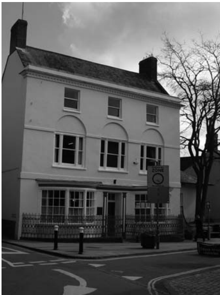
Fig.34 No.9 Cheap Street Digby Estate Office
