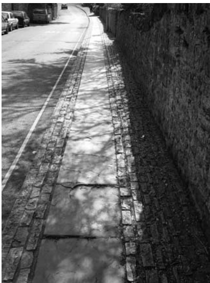
Fig.38 Traditional stone paving and sets, Hospital Lane
