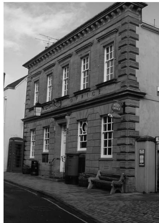
Fig.22 Post Office, Cheap Street
