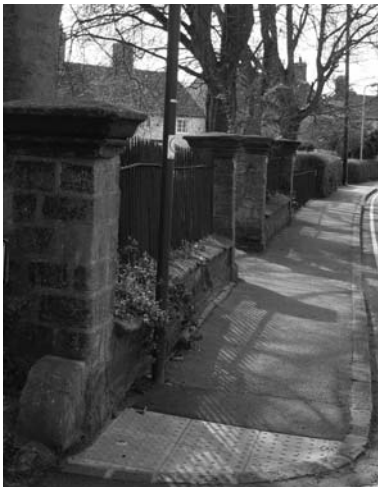
Fig.74 Westbury walls and piers
