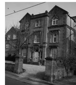
Fig.71 Saffron Court, The Avenue
