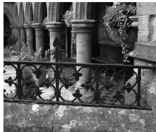
Fig.13 SS. John Almshouse (detail)
