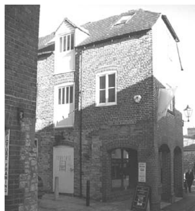
Fig 44. Former warehouses in Durngate St
