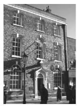
Fig 70. Barclays Bank in South Street with a splendid combination of vitrified and rubbed and gauged brickwork
