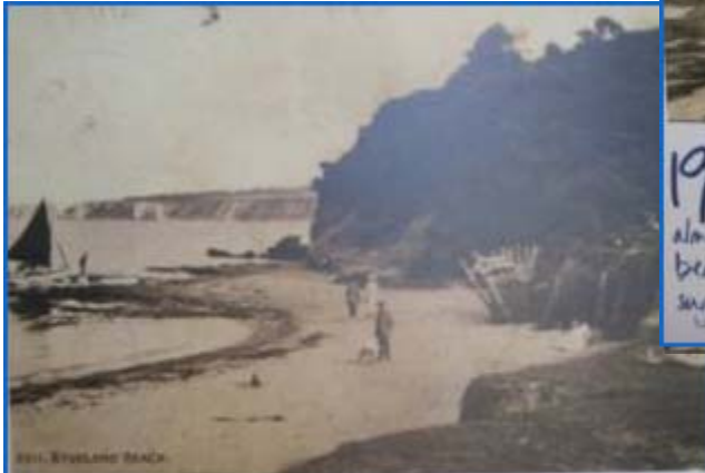
1927. There is a distinct drop between dunes and sea shore in this view, where the tidal action has carried material away. You can see some tidal defence timber work in a bad state of repair.
