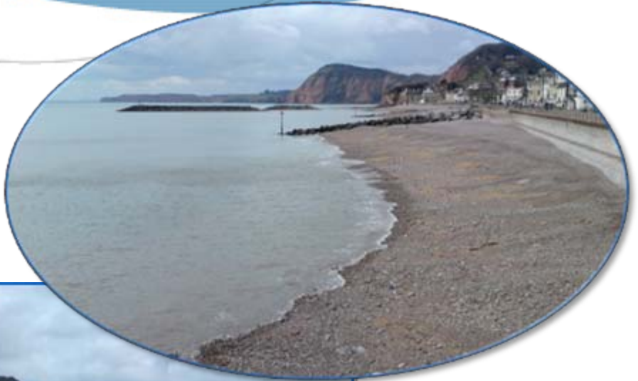
Exposed shingle beach with two small offshore breakwaters at the west end.
