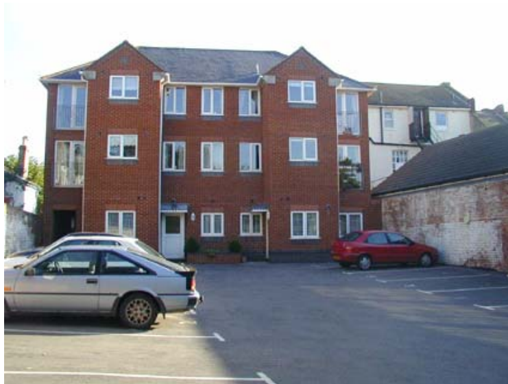
Housing Development adjacent to the Magistrates Court Site
