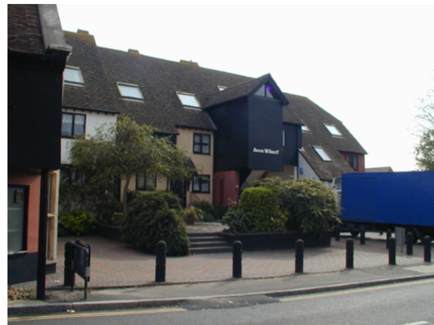
Front elevation, Avon Wharf
