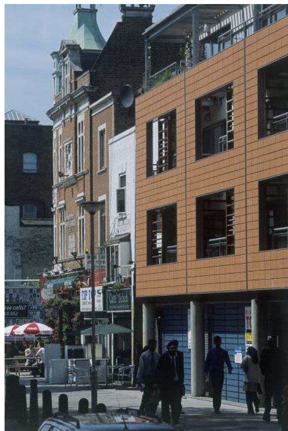
Integrating with adjacent building/ left
