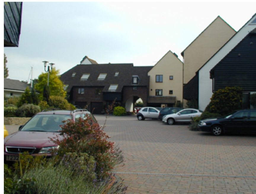
Rear courtyard, Avon Wharf
