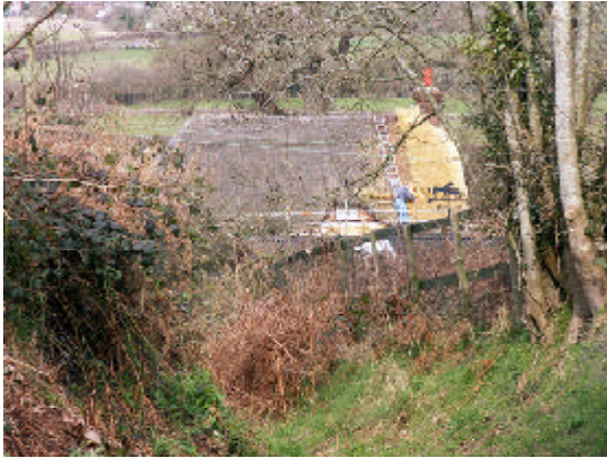
431 Long Lane viewed from Merrifield
