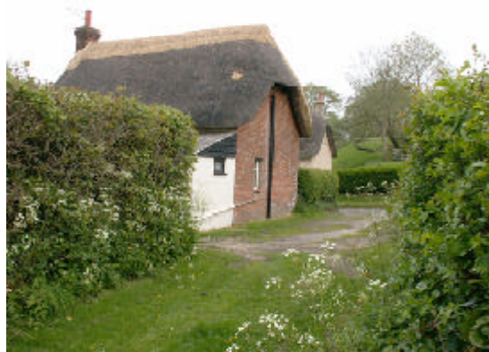
Rear of 431 Long Lane
