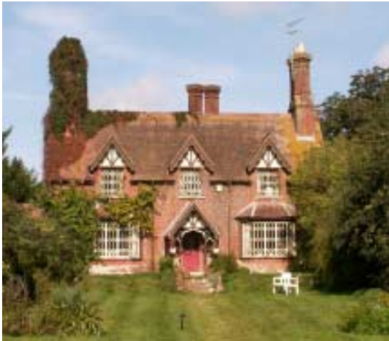
The old schoolhouse, a Grade II Listed Building
