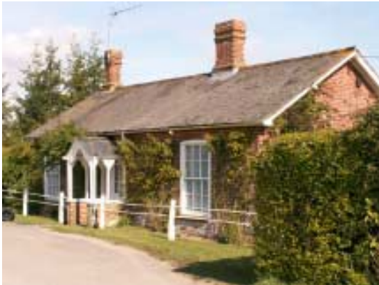
Turn of the century Estate houses in Park Lane
