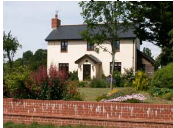
New house south west of Forge Cottage
