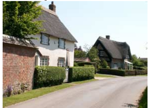
School Cottage & No.198 West Street, both Grade II listed buildings
