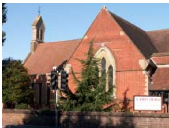
South front of St. Johns Church
