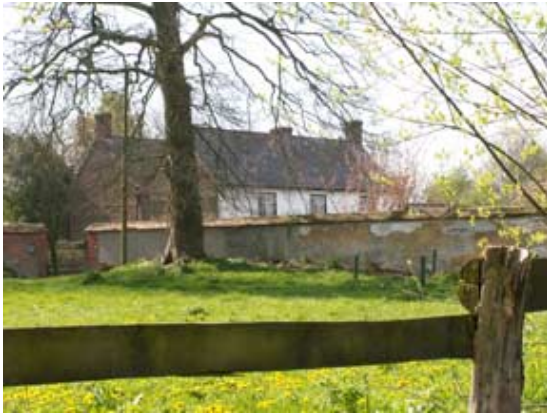
Manor Farmhouse, a Grade II listed building
