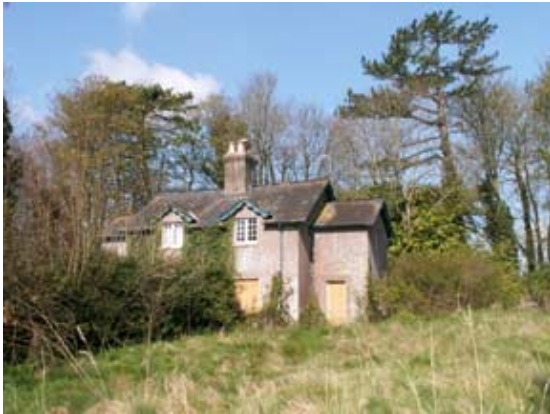
Former estate house near Butler's Barn
