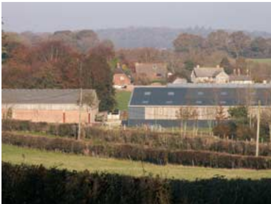
The barns at Manor Farm
