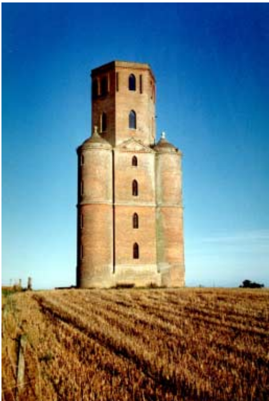
Horton Tower, a Grade II* listed building is a prominent landmark now used as a telecommunications relay tower
