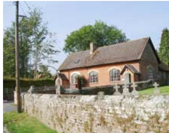
Old School House & Village Hall (Grade II Listed Building)
