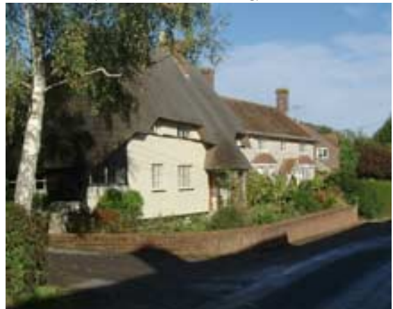
Old Timbers (Grade II Listed Building)
