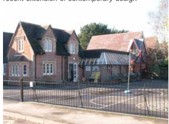
Hampreston CE VA School a 19th C building with recent extension of contemporary design
