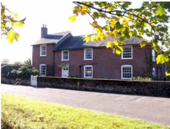
Manor Farmhouse, a Grade II Listed Building
