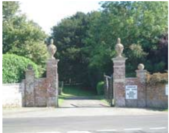
West entrance to Edmondsham Park
