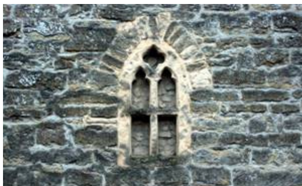
Figure 164: Detail of 14 th century window reused in Emerenciana, Nethercoombe
