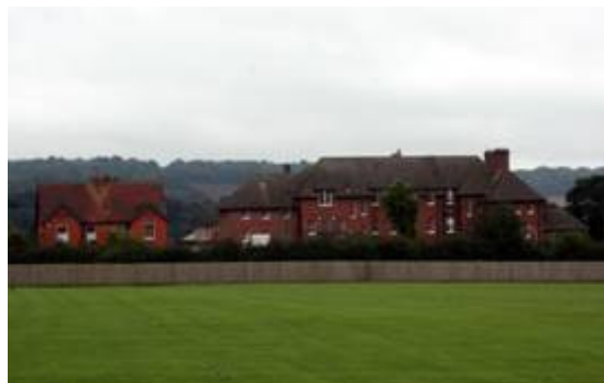
Figure 145: Lyon House (Sherborne School) and 13-15 Richmond Road
