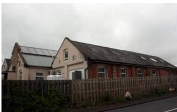
Figure 149: Former print works, Yeovil Road
