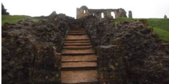
Figure 126: Sherborne Old Castle; North Gate
