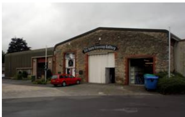
Figure 187: The Old Barn, Unit A1, South Western Business Park
