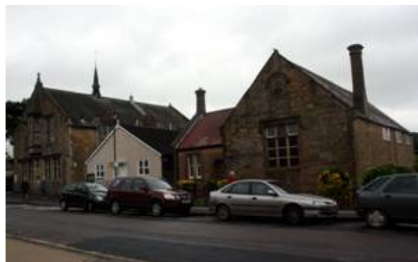
Figure 183: The Digby Memorial Church Hall (left) and Masonic Lodge (right), Digby Road
