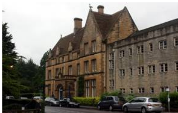
Figure 182: The Digby, formerly the Digby Hotel
