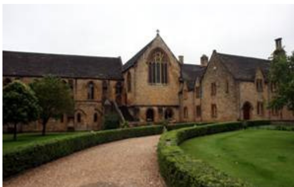
Figure 37: Sherborne School Library (left), Chapel and School House Studies (right); formerly the abbot's kitchen
