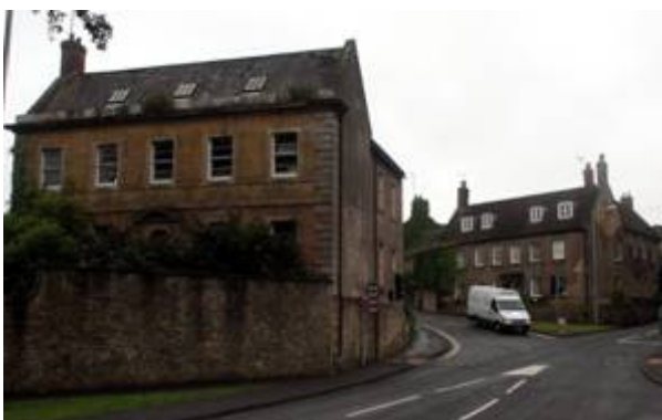
Figure 39: Newell House (left foreground) and Kitt Hill House (right background)
