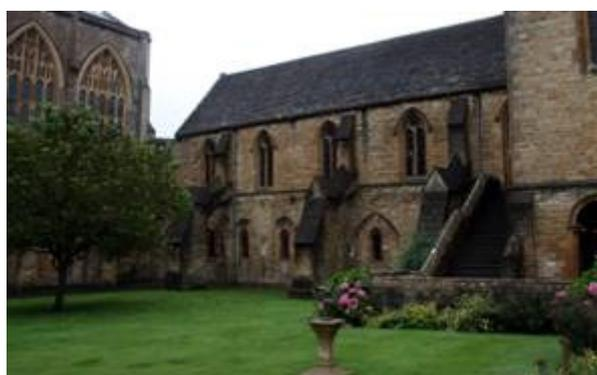
Figure 23: Sherborne School Library showing the remains of pilasters and vaulting from the lost west cloister walk
