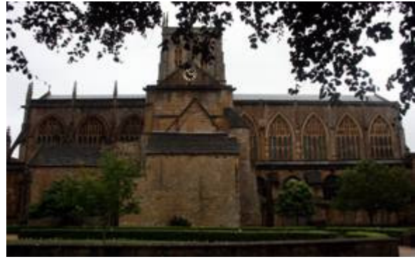
Figure 13: The north front of Sherborne Abbey showing The Slype and successive gable scars from the Abbey cloisters on the external wall of the north transept
