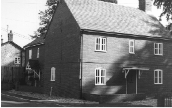
Simple house types are cheaper to build, allowing more to be invested in good quality materials. These recent houses having plain clay tiles and stock bricks, harmonise with other buildings in Cranborne, but might look out of place in, say, Shapwick.
