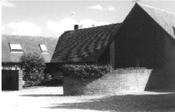
Manor Farm, in the centre of Hinton Martell, has been partly reconstructed and converted into five dwellings. A modern architectural treatment has been adopted but its traditional form and materials were retained.
