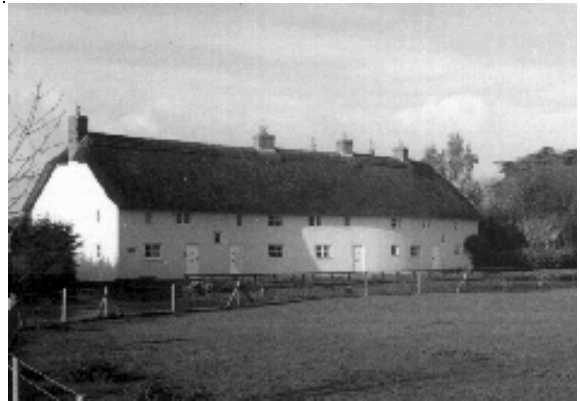
A row of rendered and thatched cottages, constructed in 1988 at the northern end of Sturminster Marshall, relate in form and materials to a similar row adjacent to the church. These cottages, which replaced a single inter-war bungalow, make a positive contribution to the character of the conservation area. The gentle curves in the cottage walls belie their concrete block construction.
