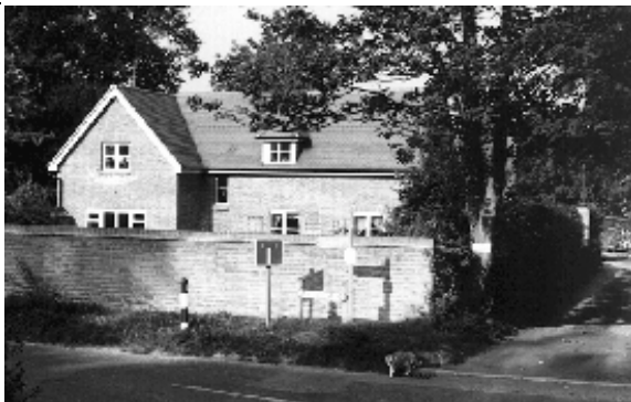
A recent house in Gussage St. Michael having low eaves height, a narrow building span and 45° roof pitch. The size and disposition of windows ensure that solid areas, both walls and roof, remain dominant.
