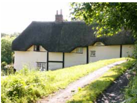
18 th C plastered cob cottage in Pamphill.
