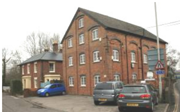
Figure 51: Walford Mill House and adjoining industrial buildings
