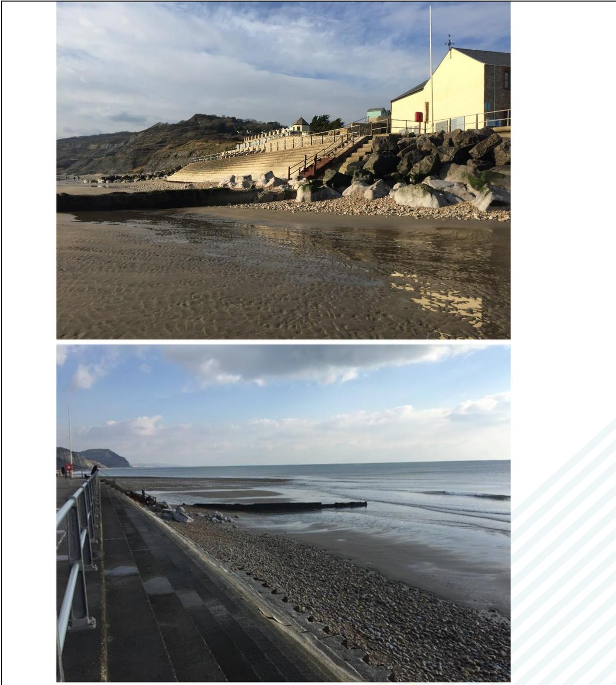
**Figure 2-7 Coastal defences to west of River Char showing stepped revetment with exposed sheet pile toe in places and placed rock for additional protection**
