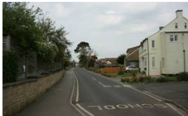
Figure 39: View up Lower Sea Lane towards the Street.
