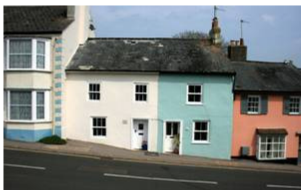
Figure 20: Charm Cottage and Heron Cottage, formerly a cottage hospital.
