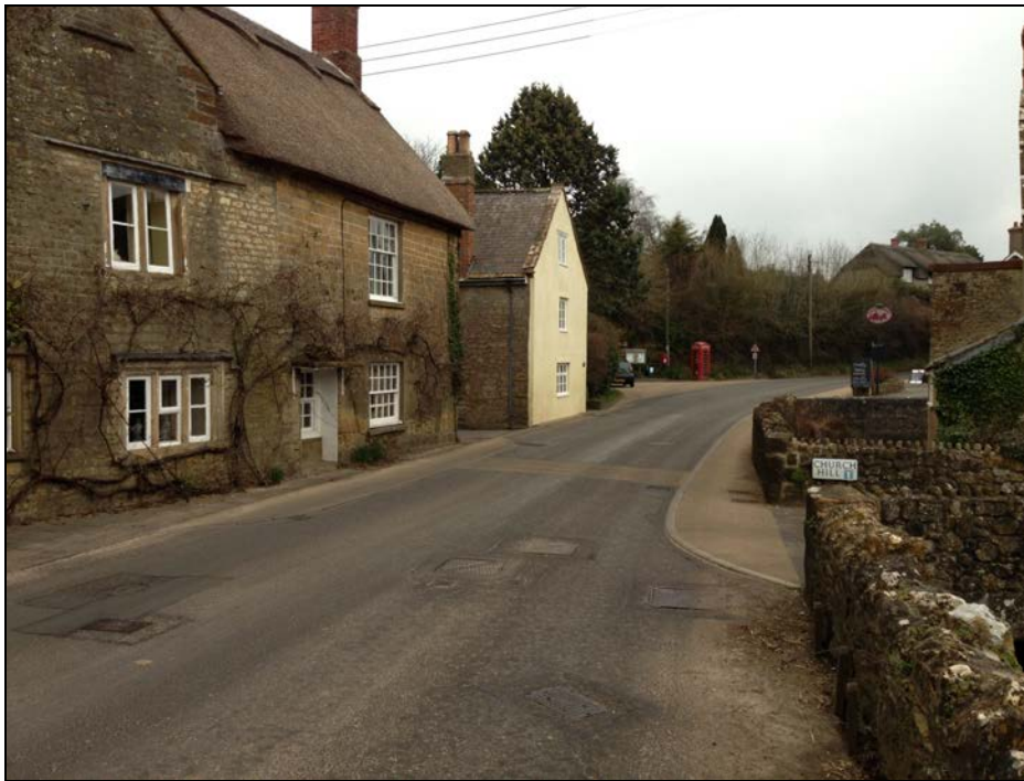
Photo 1: Dropped Kerb Footway Arrangement on the A356 through South Perrott
