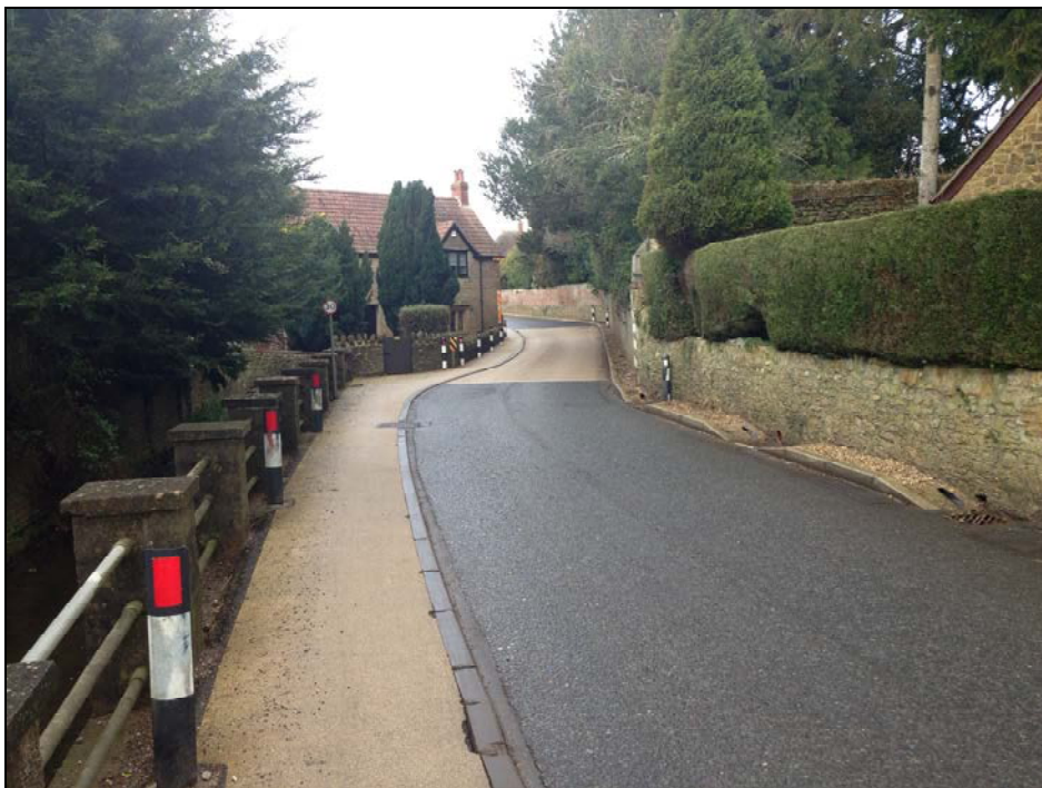
Photo 2: Dropped Kerb Footway Arrangement on the A356 through South Perrott
