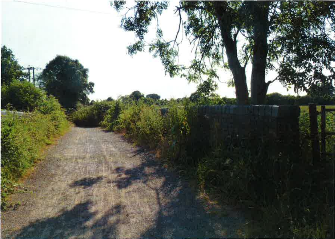
Figure 7.17: Ward’s Drove Bridge, looking south-west along Ward’s Drove
