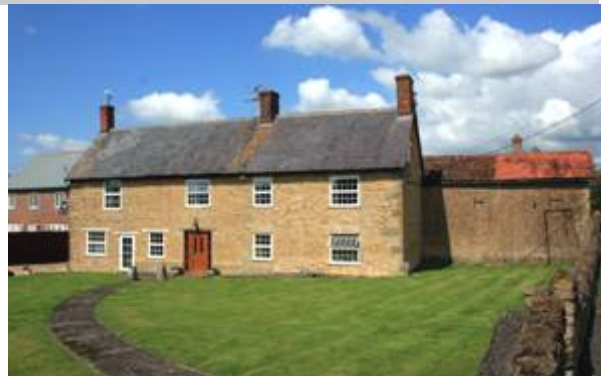
Figure 84: Peacemars Farm House and attached outbuilding, with modern housing to the rear (left).
