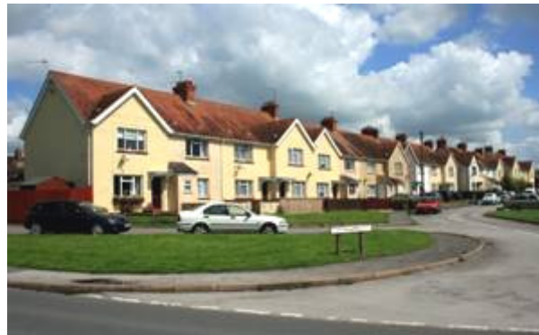
Figure 86: View east along Lodbourne Terrace.
