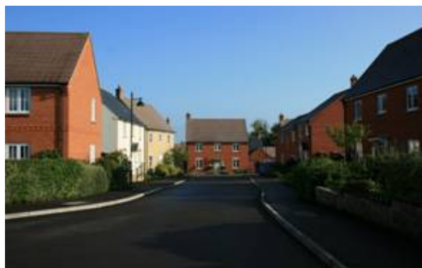
Figure 35: Barnaby Mead Housing Estate.
