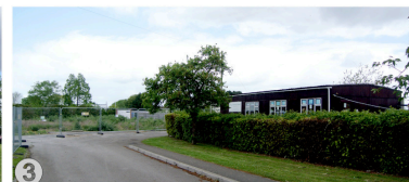
3 Nursery viewed from the existing site entrance
