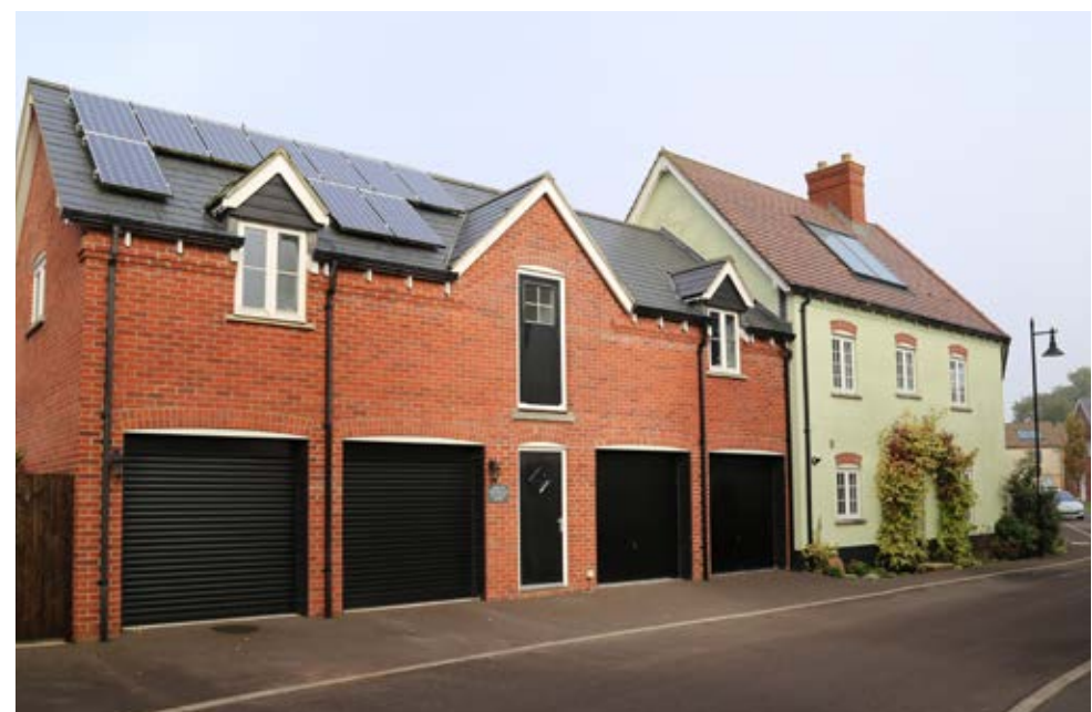
Recent housing development Gower Road. This development has attempted to reference the local vernacular, however there are issues with scale and density.
