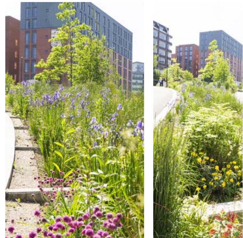
Example of Sustainable Urban Drainage System in Sheffield City Centre
