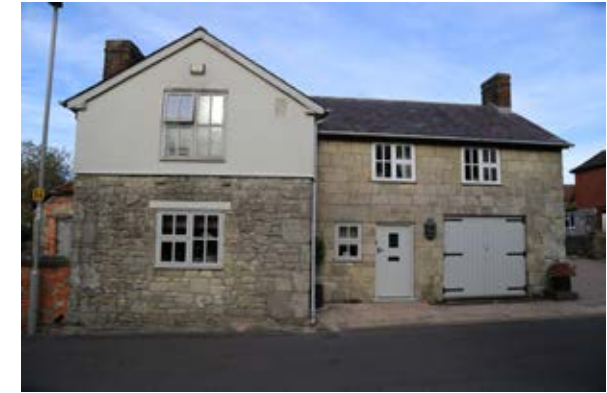
Contemporary renovation Haines Lane
