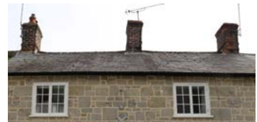
Chimney detailing found in Shaftesbury
