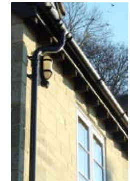
Classic half round gutter with round downpipes and traditional brackets in cast iron effect finish; hoppers can be varied but should allow for high capacity drainage
