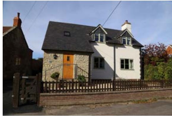
Contemporary renovation Well Lane
