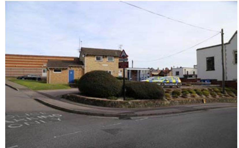
20th Century Police Station building
