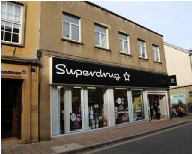
Poor quality shopfront High Street
