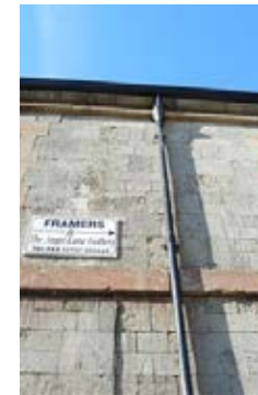
Classic half round gutter with round downpipes and traditional brackets in cast iron effect finish; hoppers can be varied but should allow for high capacity drainage
