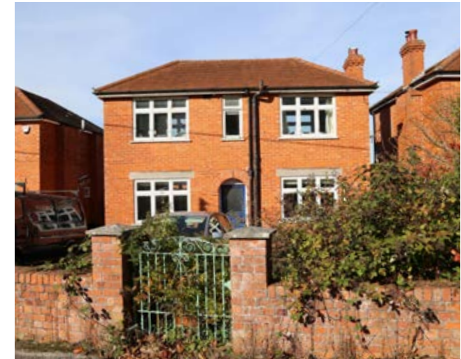
Post war property, Breach Lane
