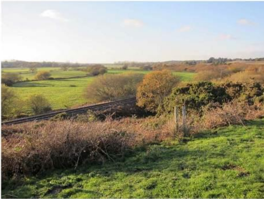
Photo 4: The Swanage Railway passing through a gorse scrub lined cutting.
